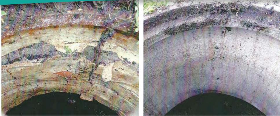
Manhole needing repair with a failed liner on and the same manhole one year after rehabilitation with calcium aluminate cement.
