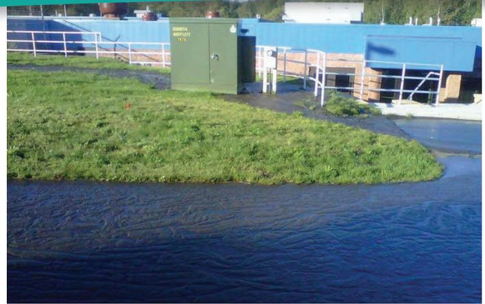
An example of an extreme case of anaerobic digestion foaming that runs into roadway, parking lot, and walkway.
