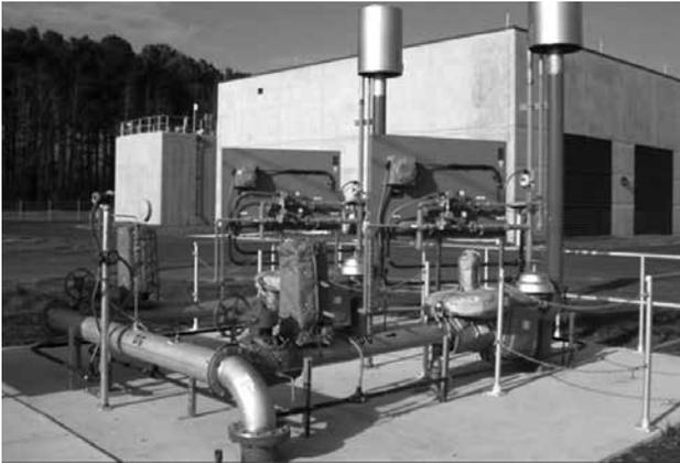
Unconfined “candlestick” flares can be a source of methane when combustion of biogas is done under suboptimal (windy) conditions.
