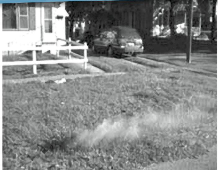
Lateral inspection using smoke testing.
