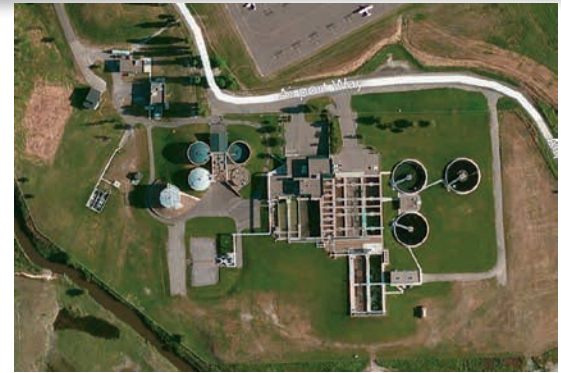
Aerial photo of the City of Kalispell, Montana Advanced Wastewater Treatment & Biological Nutrient Removal Facility, one of the facilities that participated in the study.
