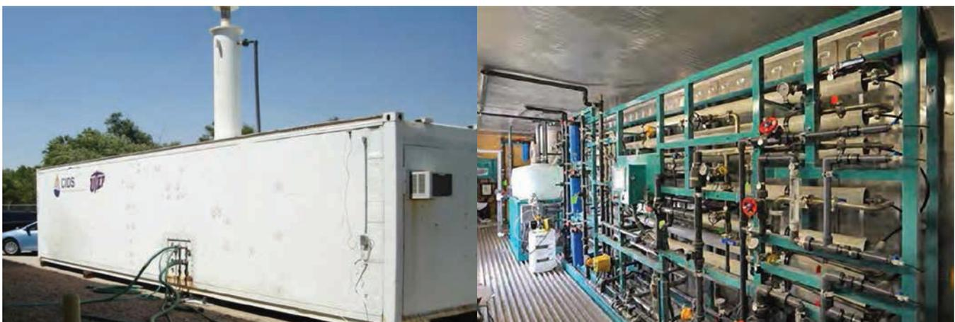
Containerized nanofiltration unit in position outside the La Junta Plant (left). Interior view of the nanofiltration unit (right).
