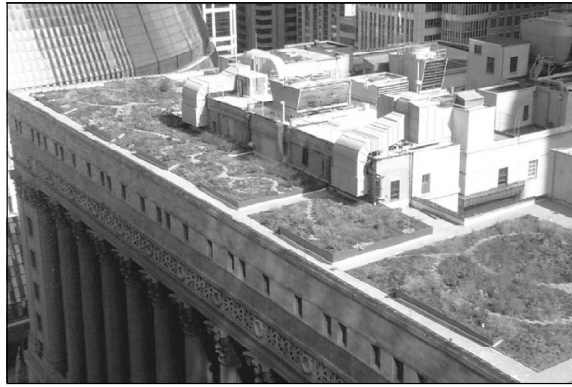
Chicago's first green roof, atop City Hall.
